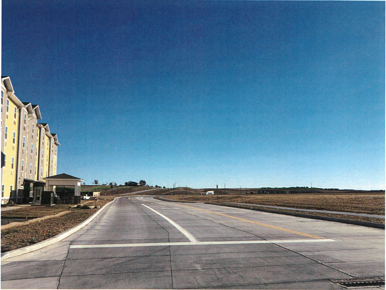
Completed road within Fox Hills Village
